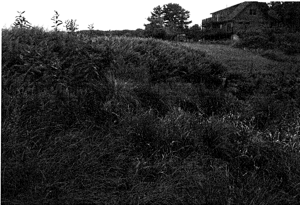
Photo 4 Dam ID# 163-0188 Treasure Lake Dam 08/10/2023 Downstream Embankment View: Center of dam
