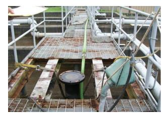
A walkway over an oxidation ditch is in disrepair.
