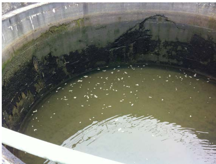
Post Equalization Tank
