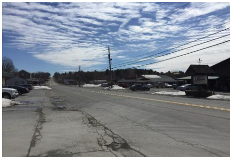
Lower East Broadway features areas of uncontrolled access that lack adequate curb and landscape separation between parking areas and the road, which also creates an inhospitable pedestrian environment.
