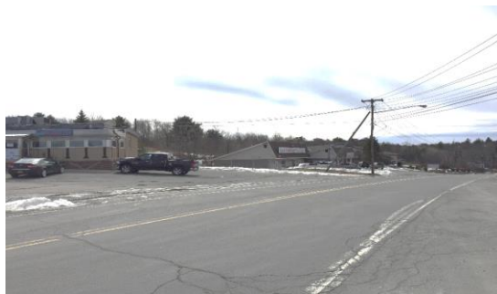
An example of uncontrolled access to the road corridor. Note the lack of curbs, sidewalks, and landscaping that create an unsafe and uninviting pedestrian environment.
